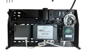
**Ligero** – On site compact Energy Management System that is rack or wall mountable in the building communications room. Full load balancing and energy tracking Intelligent OCPP
